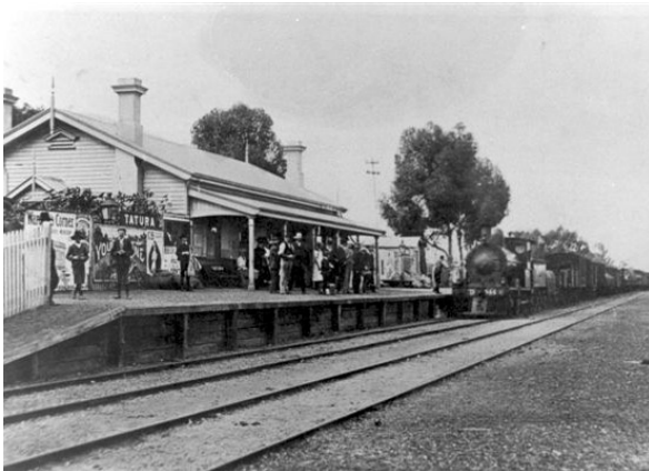
Former Tatura Railway Station.
